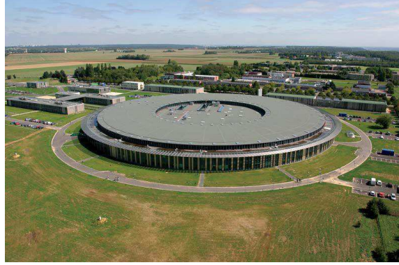
Figure 2.20: Picture of the SOLEIL synchrotron [65].
