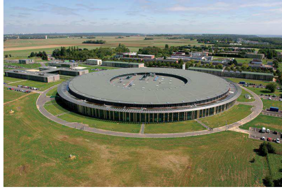
Figure 2.20: Picture of the SOLEIL synchrotron [65].
